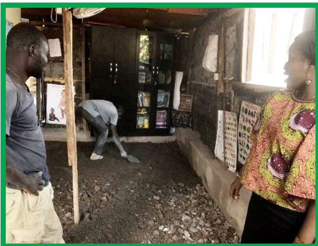
Renovation of the old classrooms
