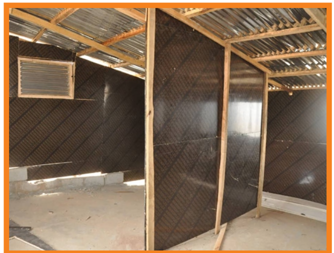
Interior of the two new classrooms
